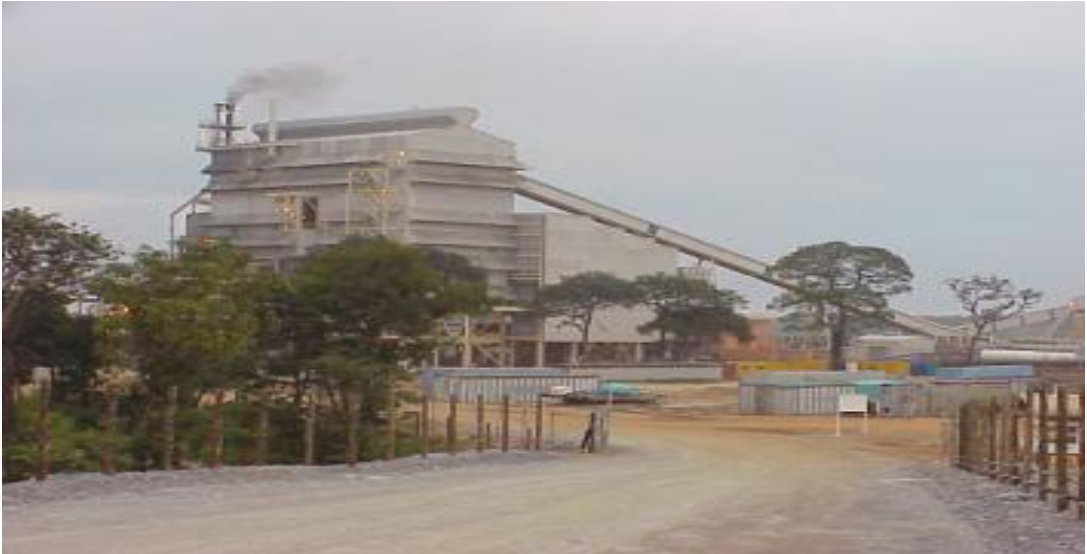
Figure 2: Chambishi Metals 40 MW DC Arc Smelter
